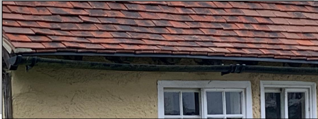
Poorly fitted gutter on north elevation
